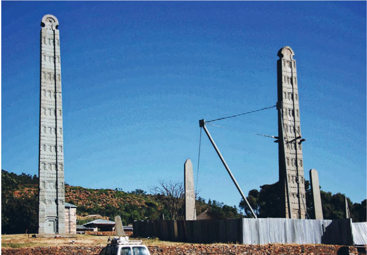
Fig. 8. Stela 2 and Stela 3 at Aksum in 2009. Stela 2 is reerected in its original position to the left in the photograph. Stela 3, now slightly unstable, is balanced with a counterweight. Photo Ib Friis.
